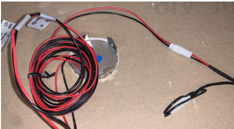
Connet the driver Whit multipull fixture use a splitter
